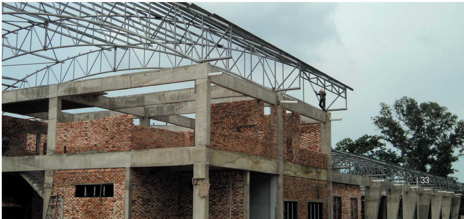
Figure 3 Exis Tech’s New Factory (under construction)
