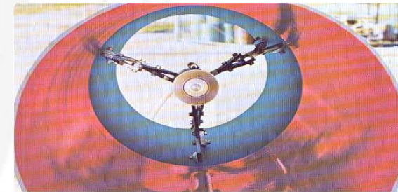
• Orbiter: coating equipment inside pipe
