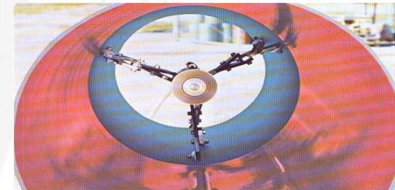
• Orbiter: coating equipment inside pipe
