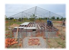
Figure 26: Lay the Heated Floor Parts
