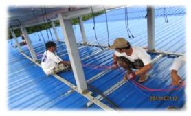
Figure 12: Panel Electrical Connection
