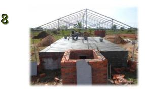
A. Lay the heated floor parts on top of the columns set up in the previous stage.
