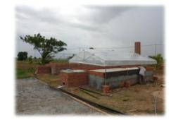
A. Plaster with mortar to prevent release of smoke from the incinerator
