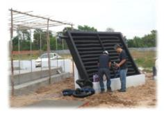
Figure 29: Set up the Solar Collector
