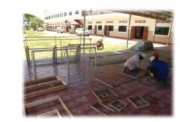
A. Weld the cylindrical pipes (diameter 4 cm) according to the dimensions (truss height 80 cm, column height 180 cm) as shown in the picture to the left.
