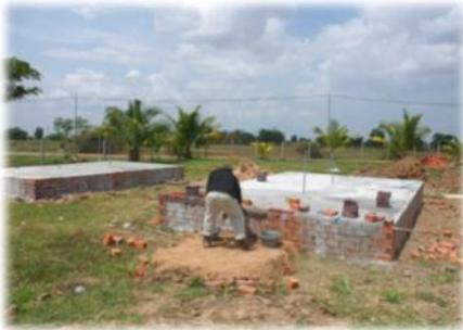
A. Place a 3 cm thick cement layer on top of the filled mud.
