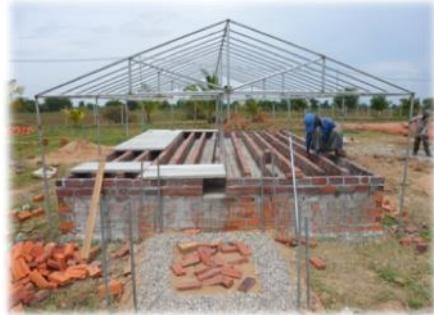
**Figure 26:** Lay the Heated Floor Parts
