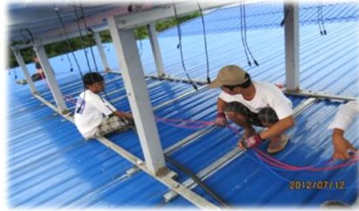
**Figure 12:** Panel Electrical Connection
