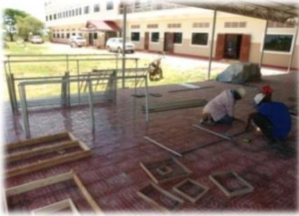
A. Weld the cylindrical pipes (diameter 4 cm) according to the dimensions (truss height 80 cm, column height 180 cm) as shown in the picture to the left.
