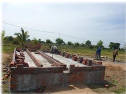
A. Block the middle part so that the smoke from the incinerator can be released equally at both ends.
