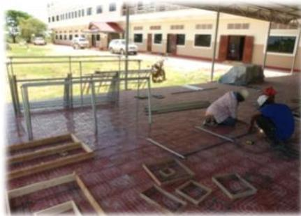
A. Weld the cylindrical pipes (diameter 4 cm) according to the dimensions (truss height 80 cm, column height 180 cm) as shown in the picture to the left.
