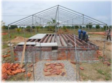
A. Lay the heated floor parts on top of the columns set up in the previous stage.
