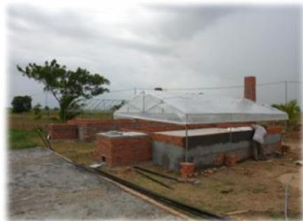
**Figure 28:** Plastering and Setting up the Plastic Sheets
