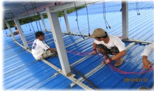
**Figure 12:** Panel Electrical Connection
