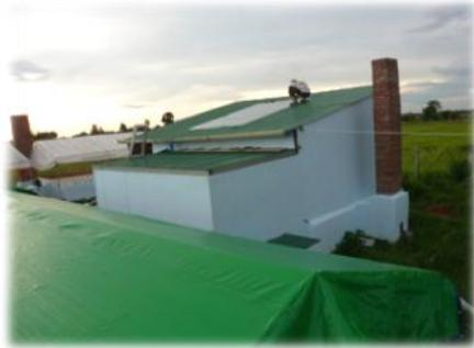
A. Install the roof on top of the masonry (height of front wall 2.8 m, height of rear wall 3.5 m), set up the solar collector in the middle and cover the surrounding with galvanized iron sheets
