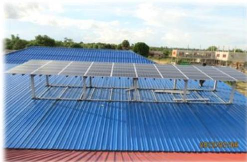
**Figure 14:** Setting up Panel Array
