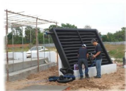
A. Install aluminum cylinders (diameter 100 mm) at 5 cm intervals within the solar collector (dimension of 2 x 3m is appropriate)
