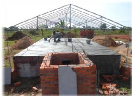
**Figure 27:** Install the Incinerator and Plaster the Heating Floor
